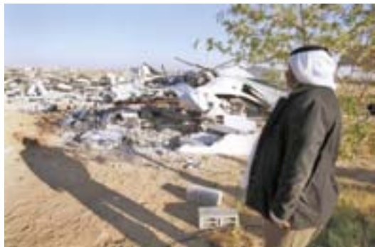
Demolished house in the unrecognized village of Bir Hadaj, February 2003 Photo by NCF
